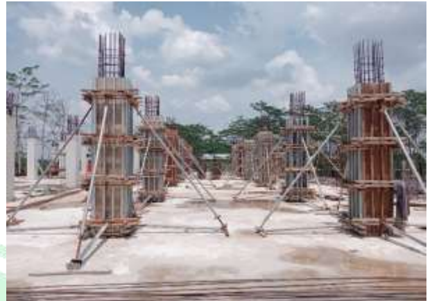
begisting Kolom Lantai 2
